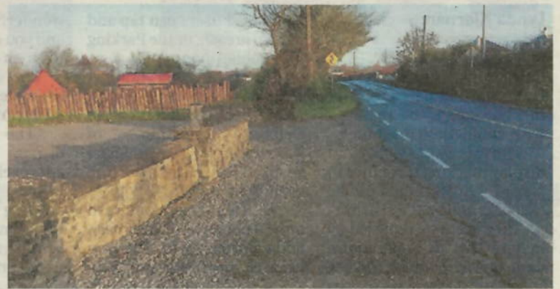
Councillors claim site is being impacted by public road
