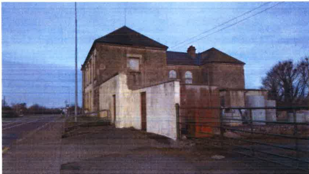
Pic.1 Derelict Courthouse Building
