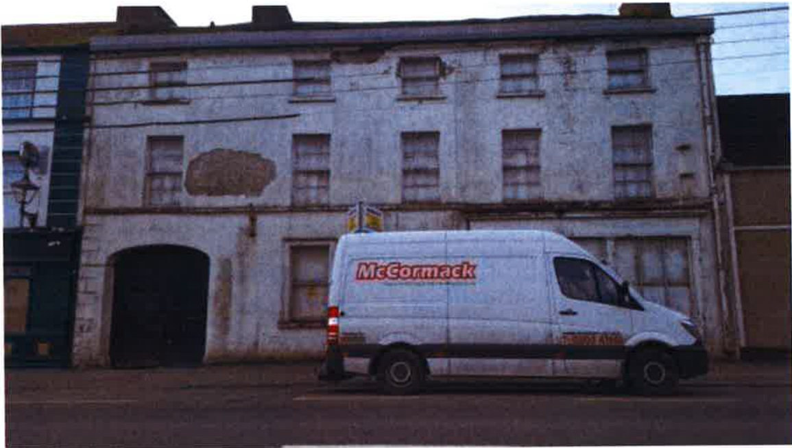
Pic.2 Derelict Property on Main Street.
