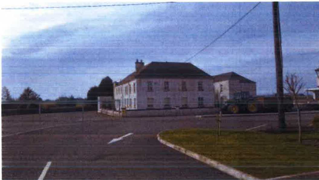
Pic. 5 Disused Convent Building adjacent to school and chapel
