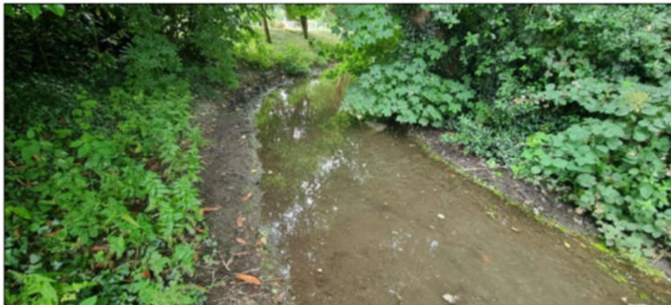
Plate 6.8 The Little Borris Stream downstream of Glendowns Pond showing gross siltation.
