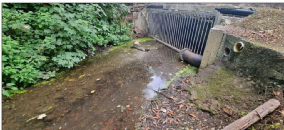
Plate 6.9 The Little Borris Stream at the culvert crossing of the Stradbally Road (N80) showing low summer flows and heavy siltation.
