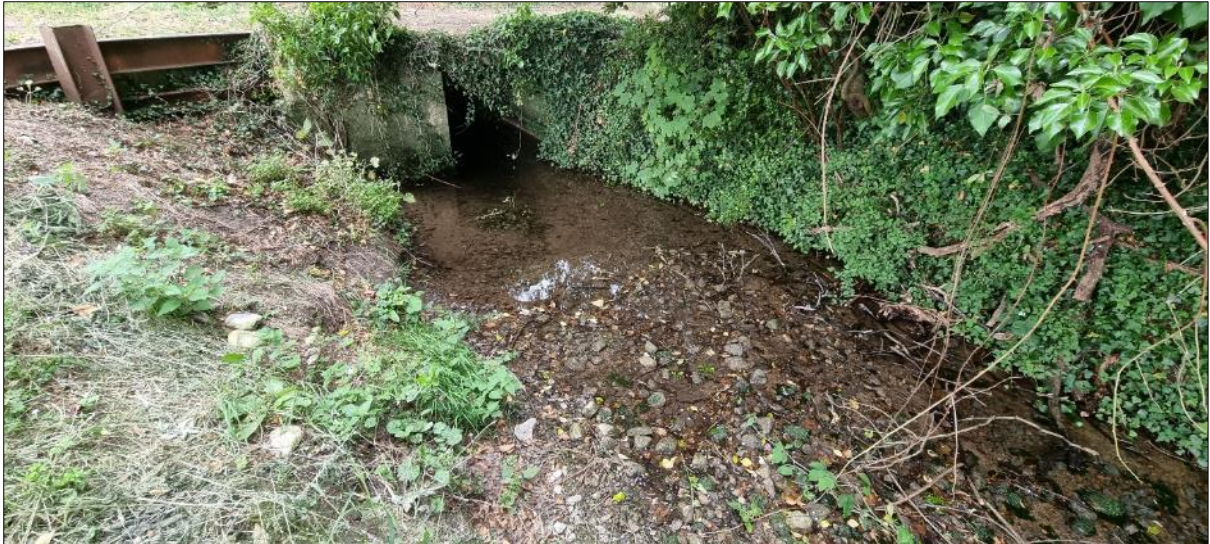
Plate 3.1 The Little Borris Stream downstream of the old bridge crossing
