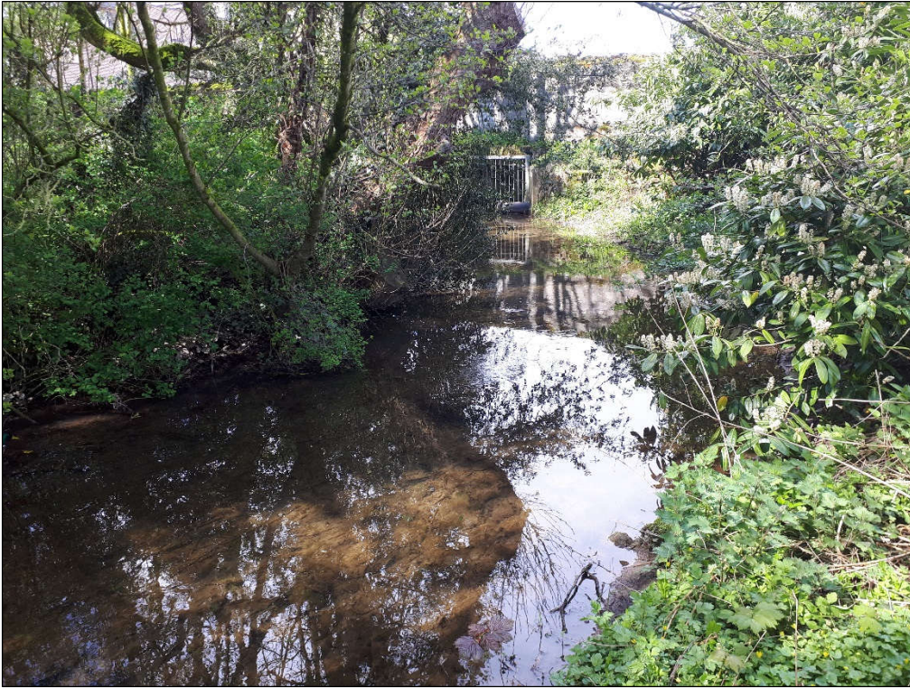
Plate 2.14 View downstream to outflow / trash screen.
