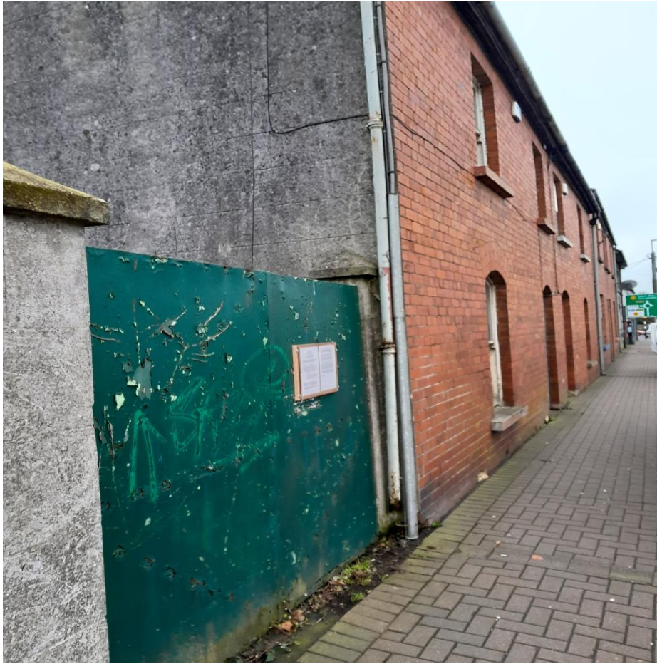
SITE NOTICE ON ABBEYLEIX ROAD, PORTLAOISE
