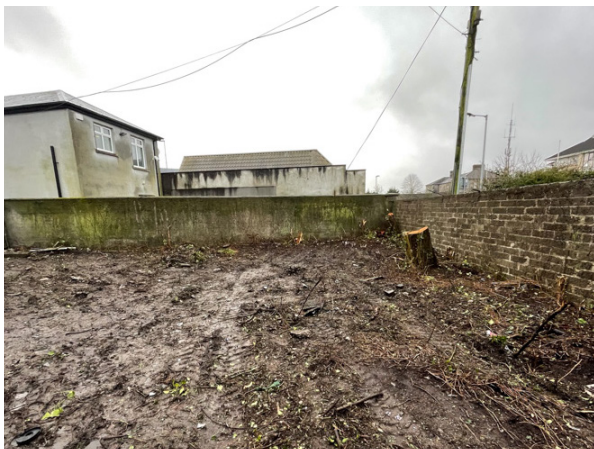
Figure 3.12 Site cleared. Showing walls to neighbouring dwelling and rear wall to Old Abbeyleix rd.
