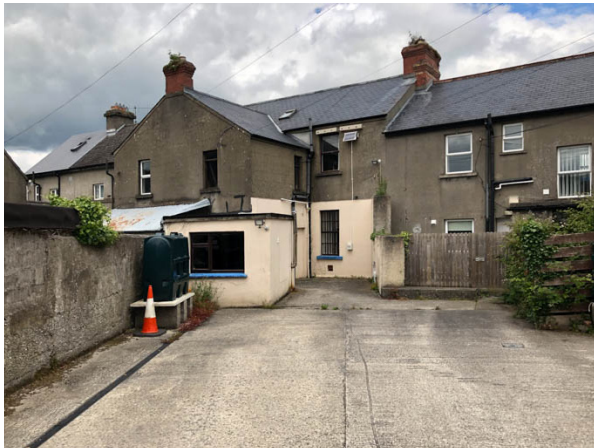
Figure 3.10 Rear of units 1 & 2.
