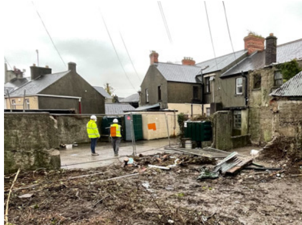
Figure 3.9 Rear of units 1 & 2. Looking from within the site.
