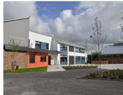
New Primary School Campus,
