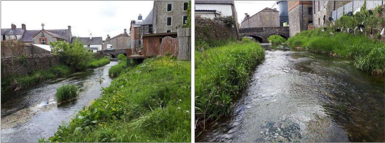
Plate 4.1 Ca. 50m downstream of N80 bridge in Stradbally (May 2021).
