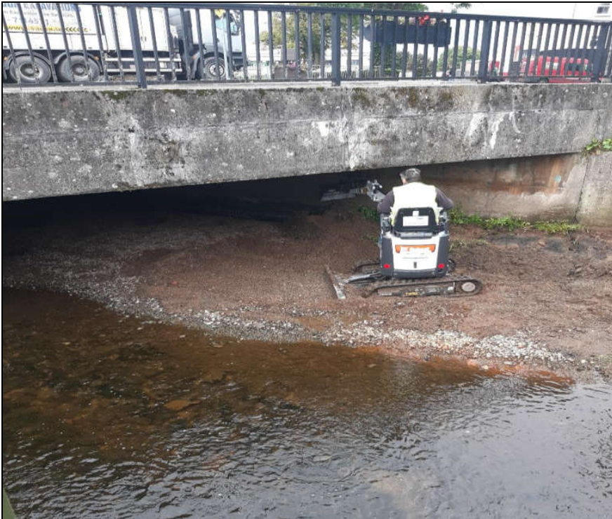
Figure 8 - It excavator feeding silt material to suction line.
