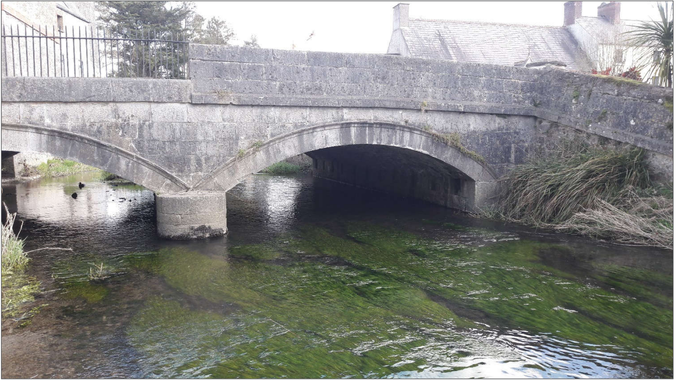
Plate 4.3 View of upstream side of the bridge (April 2022).
