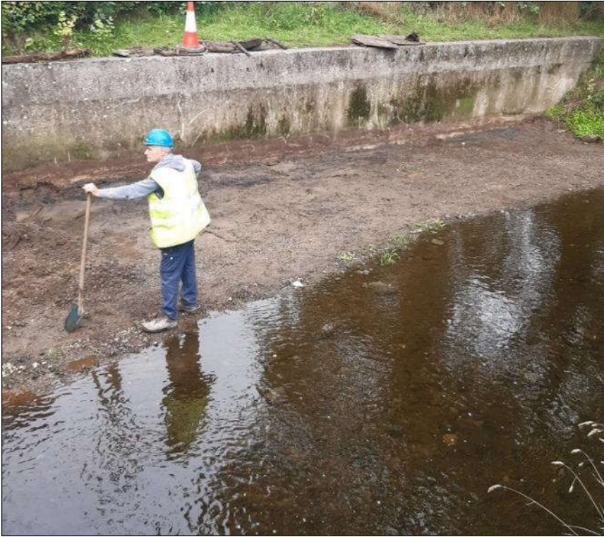
Plate 1.3 Example of similar works demonstrating how accumulated silts are only reduced at the time of works.
