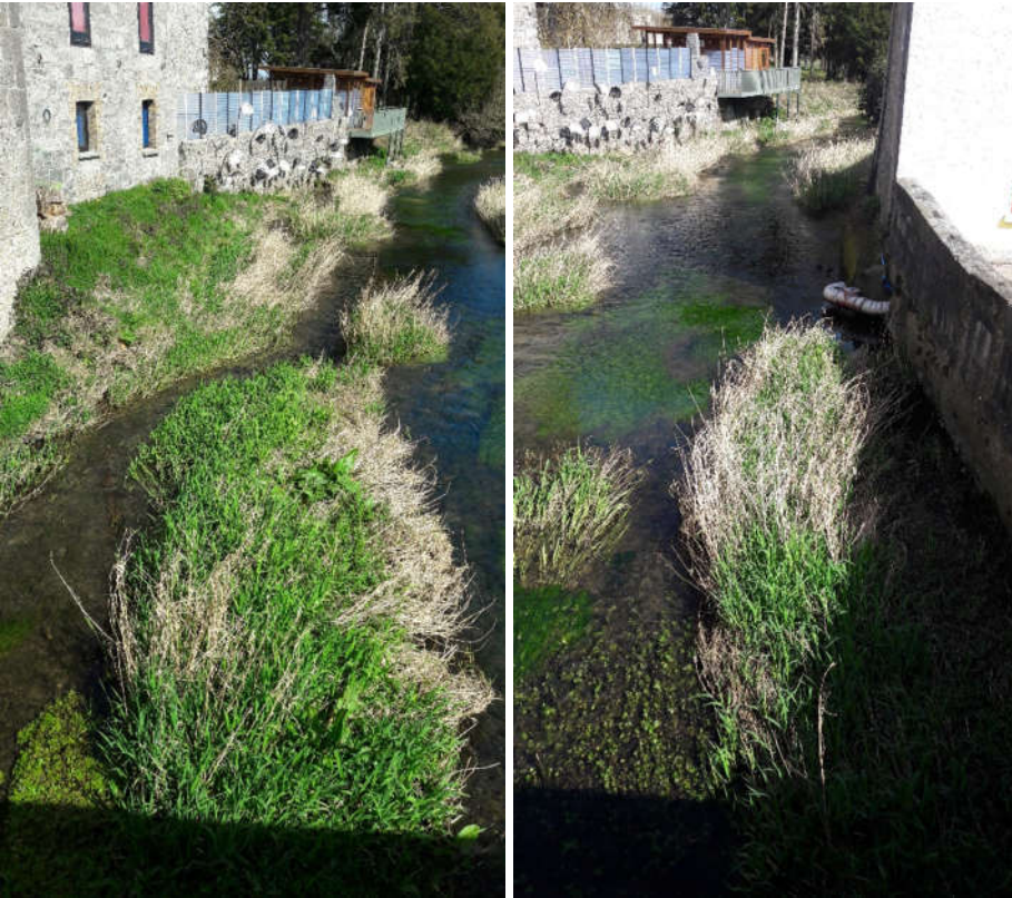
Plate 4.4 View of downstream side of the bridge (April 2022).
