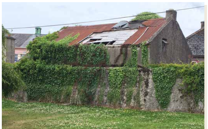
Fig. 105: Derelict building to rear seen from Laois Music Centre (Site 01)
