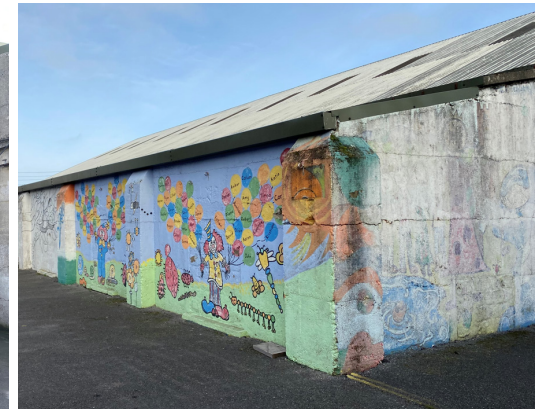
Fig.1.26: Exterior of the lean-to structure adjacent to the Granary Building
