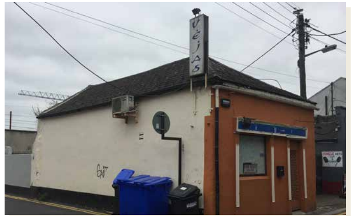
Fig.77: View from Railway Avenue. Note section of Fort wall incorporated in back wall
