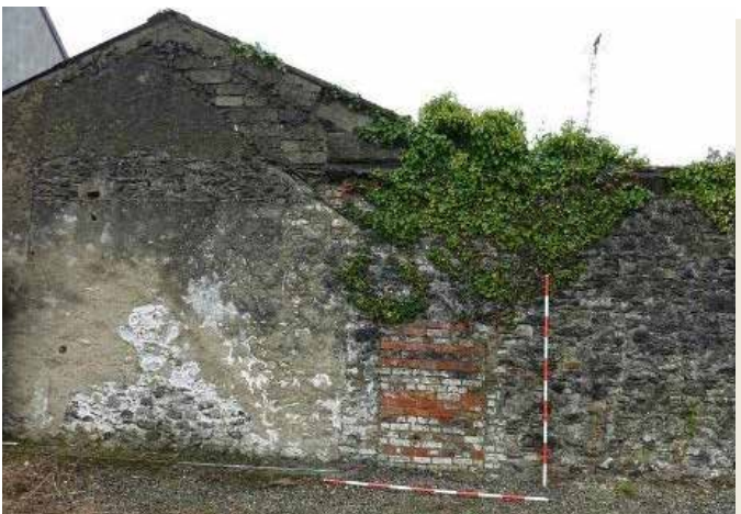
Fig. 57: Southern side of blocked-up rectangular doorway
