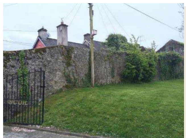
Fig. 38: South wall of Fort and internal bank
