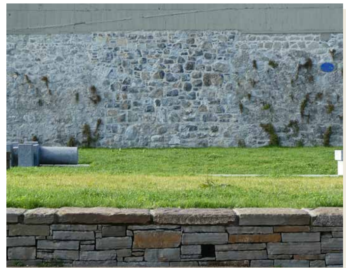
Fig. 47: Location of former doorway to mill, now blocked up externally
