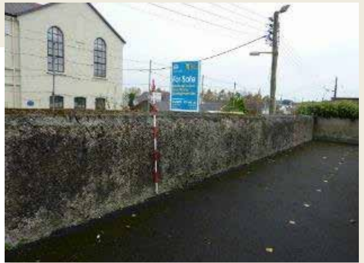
Fig. 40: Inner face of N wall
