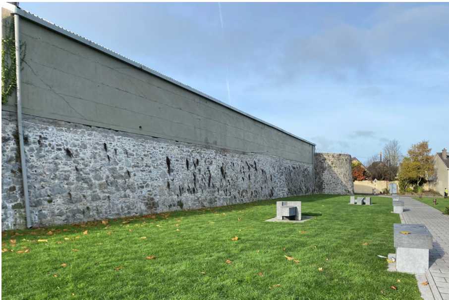
Fig.1.17: Photograph of the Eastern section of wall, along the Granary Building
