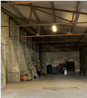
Fig.1.23: Interior of the lean-to structure adjacent to the Granary Building
