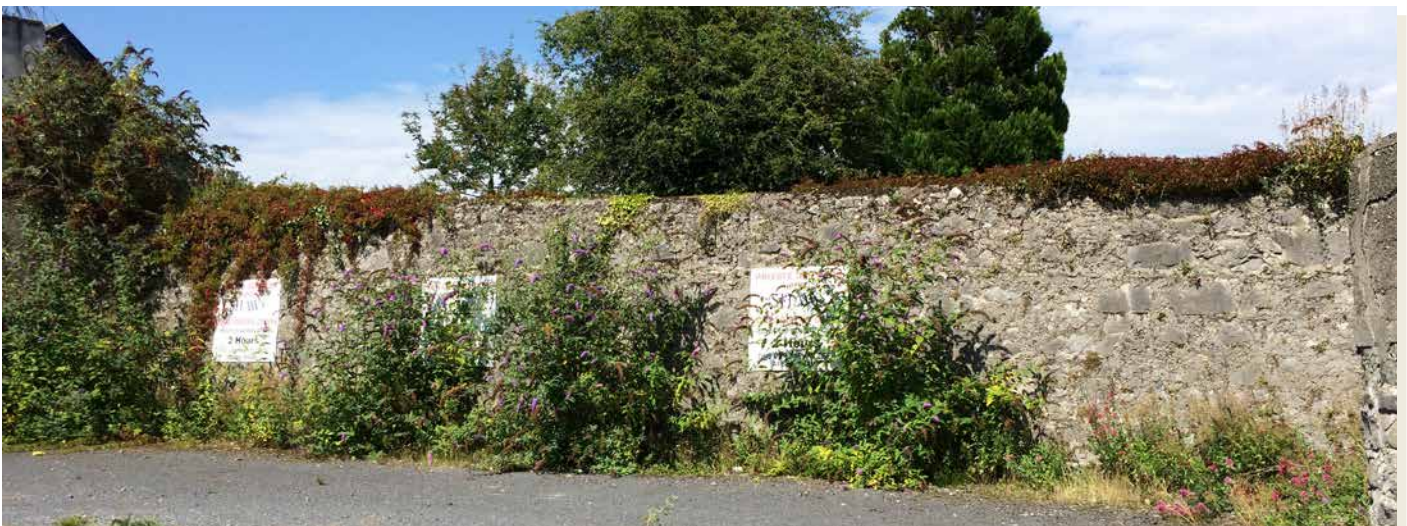
Fig. 102: Fort wall forming rear boundary of site
