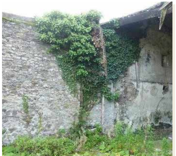
Fig. 56: South gable of western structure with blocked doorway to neighbouring Site 05
