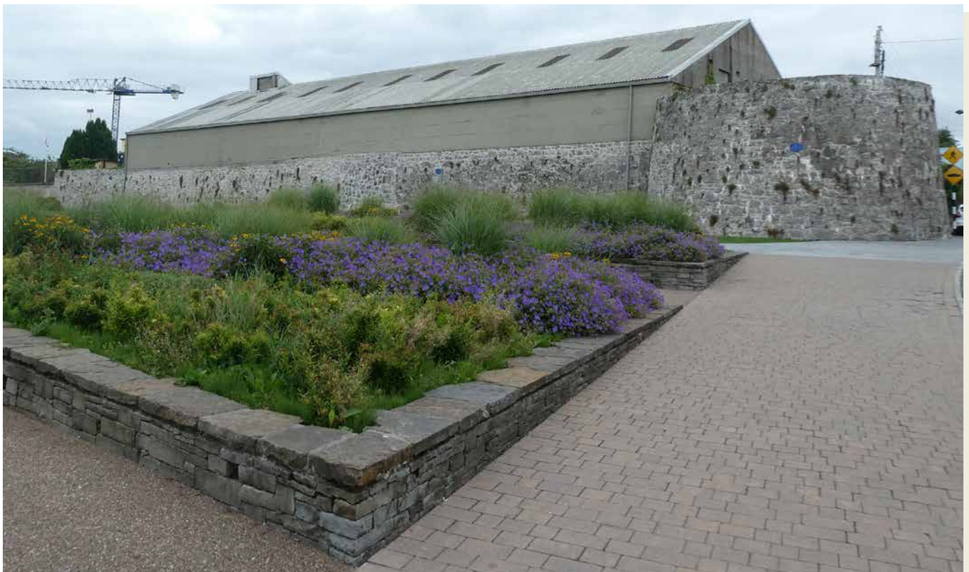
Fig. 55: West wall and corner flanker or bastion of the Fort
