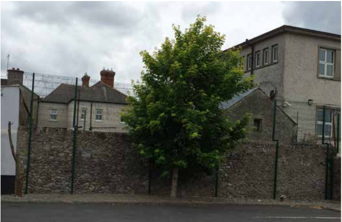
Fig. 72: Rear view from inside the Fort
