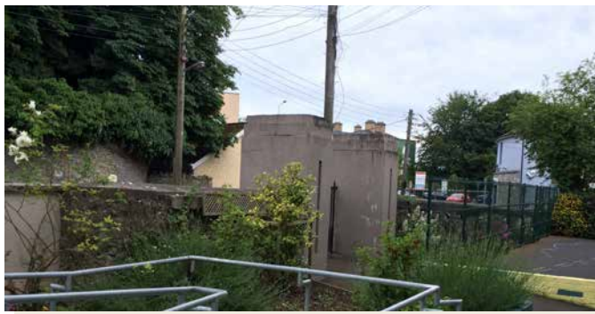
Fig. 65: Unrendered inner face of lowered Fort wall on Railway Street
