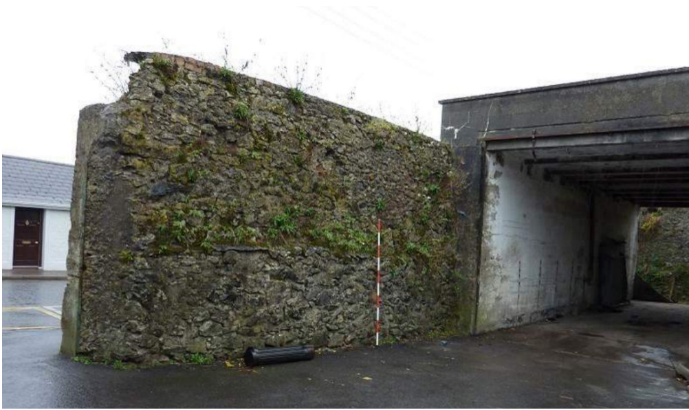
Fig.1.15: Photograph of the Northern section of wall on the internal side
