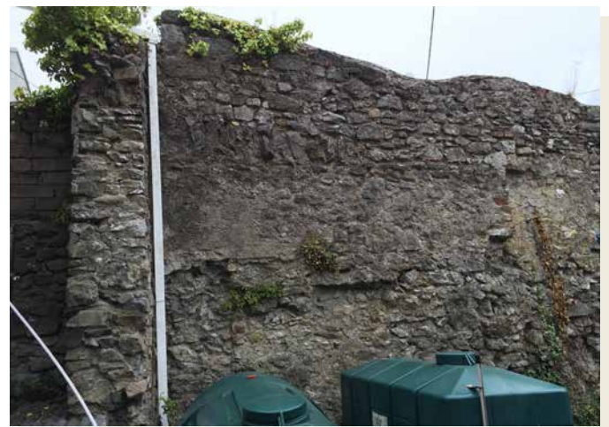
Fig. 80: Rubble stone back wall may incorporate fabric of Fort.
