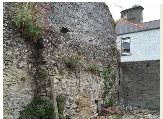
Fig. 78: Section of Fort wall incorporated in back gable
