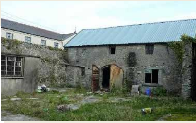
Fig. 53: Eastern structure with Fort wall to the left
