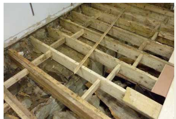
Fig. 86: View of basement in Site 13 with blocked splayed opening to left (Eoin Sullivan)
