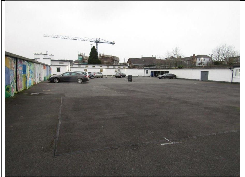
Plate 5 Showing existing tarmac yard where the temporary seats and canopy will be installed.
