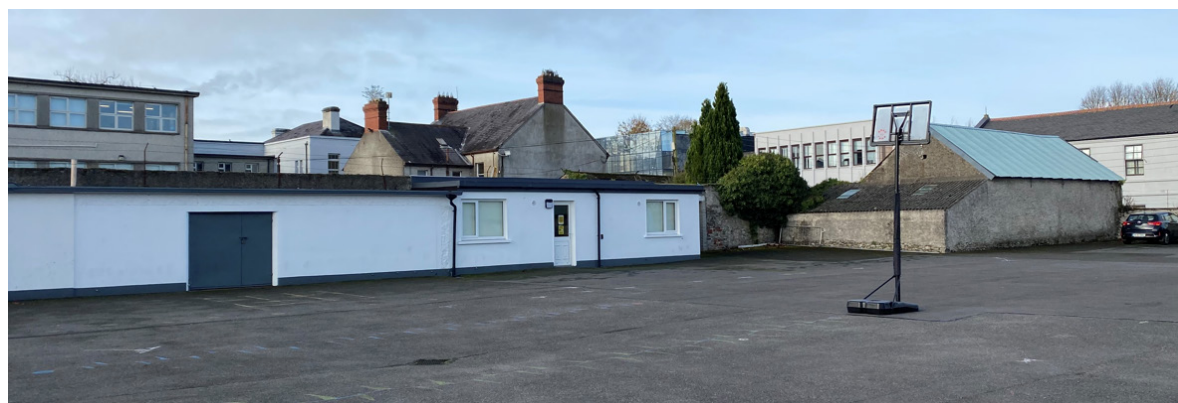
Fig.1.21: Existing school yard with Boyd Barrett shelter
