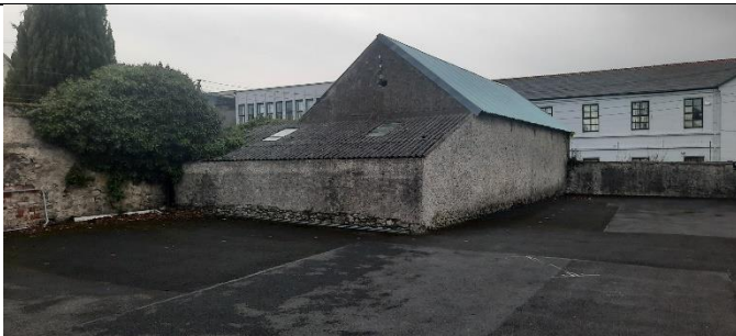
Plate 3 Showing RIC Barracks Building at northwest extent of development.
