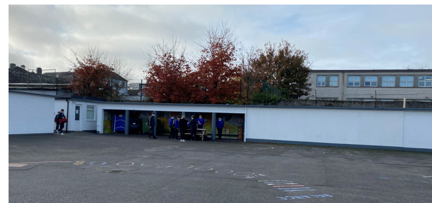
Fig.1.22: Existing school yard with Boyd Barrett shelter
