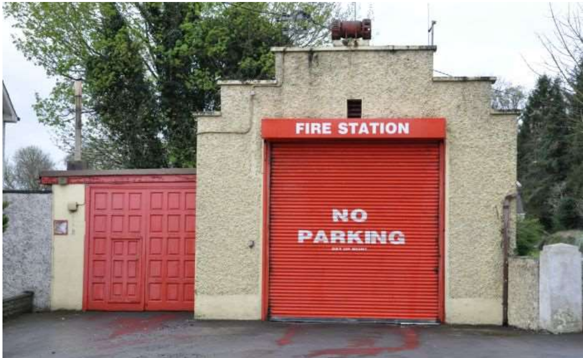
Existing Stradbally Fire Station
