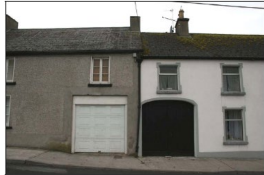
The alteration of openings and the insertion of modern doors results in slow erosion of the characteristic features of an area.
