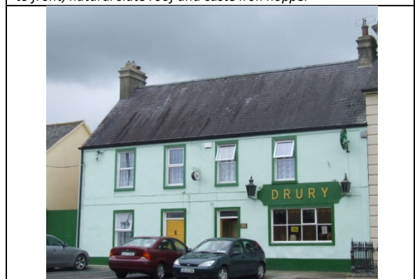
Traditional shopfront with stained glass lantern, with living quarters to the side and above
