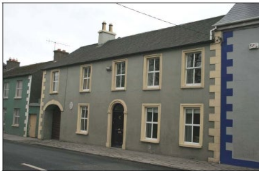
Building displaying moulded render window and door surrounds and channelled quoins, Castle Street
