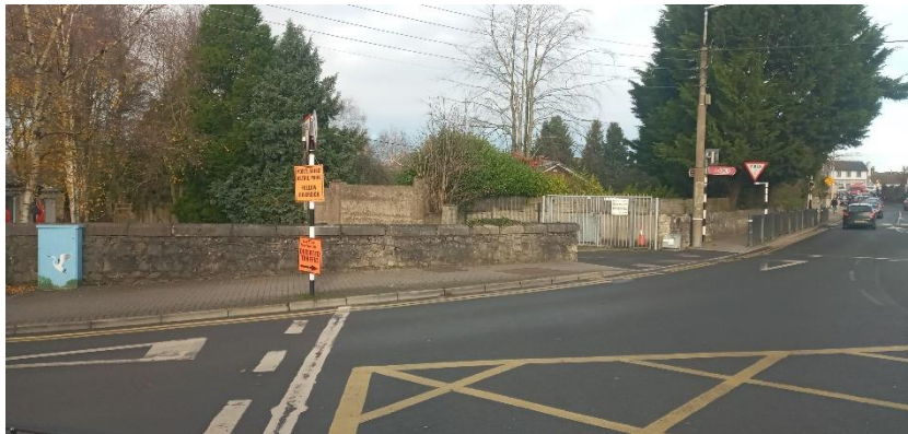
Plate 2 Bridge Street Entrance.
