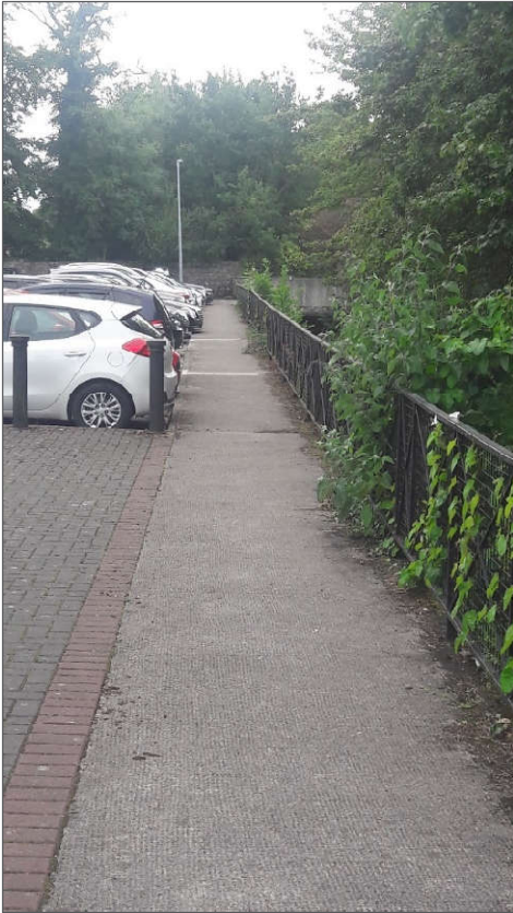
Plate 4.33 Triogue Car Park (looking south).
