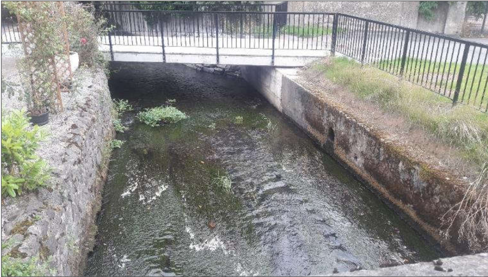
Plate 4.27 Pedestrian bridge over the River Triogue north of the N80.
