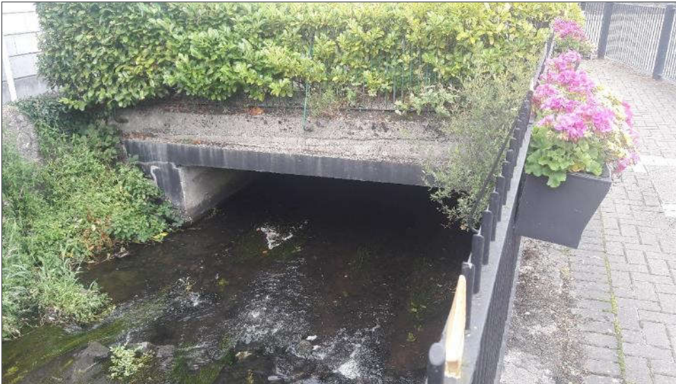
Plate 4.25 Bridge over the River Triogue at corner of N80 / Bridge Street.
