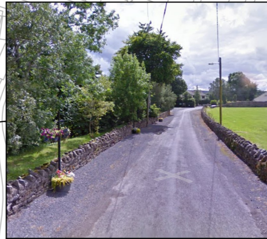
3. Access via Well Maintained Local Road
