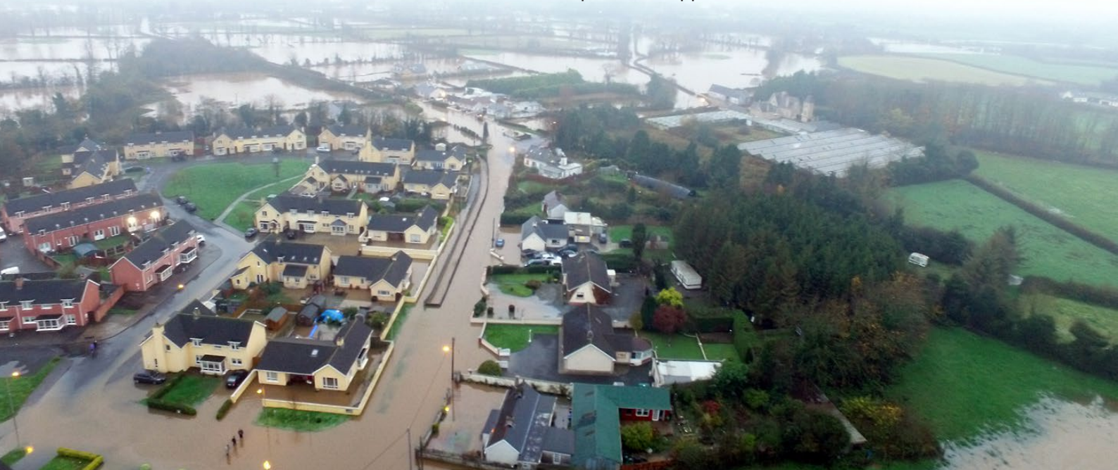
Flooding In Mountmellick in November 2017
