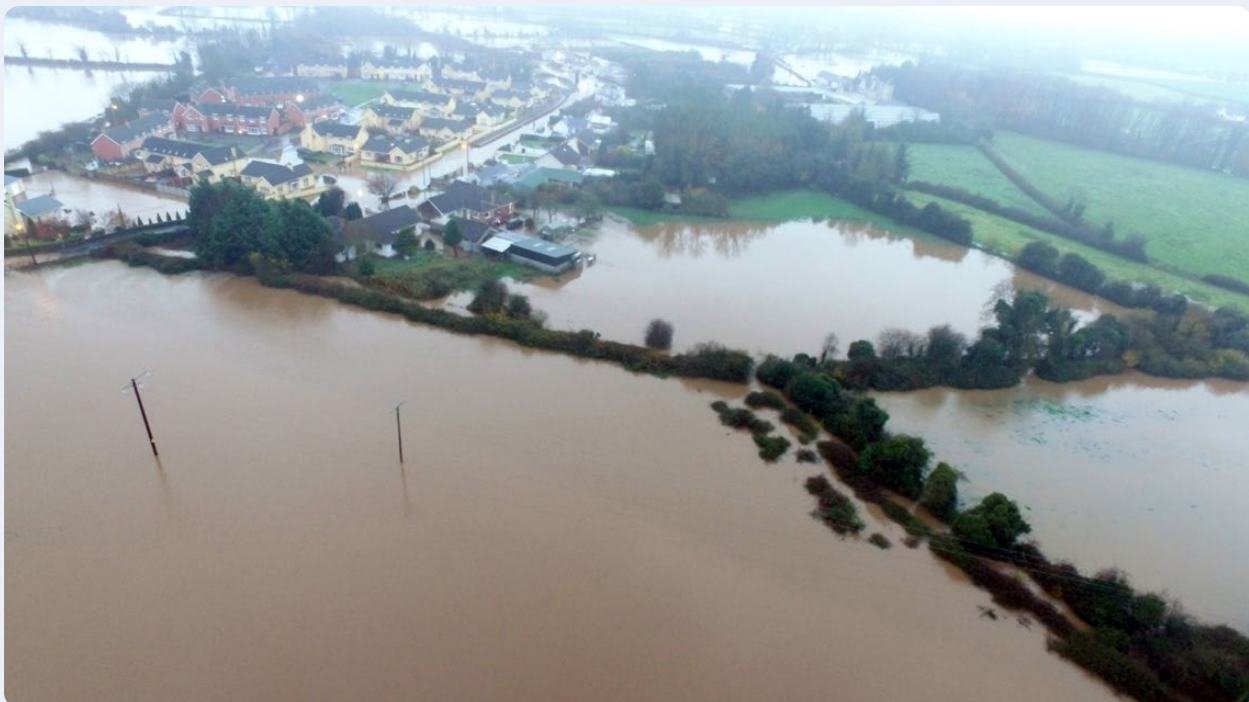
Flooding In Mountmellick in November 2017
