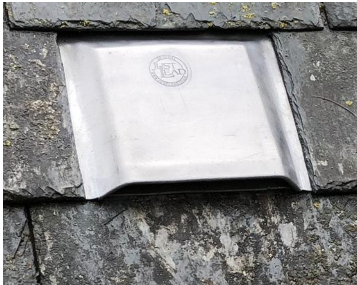
Figure 5-2 Example of lead bat tile
