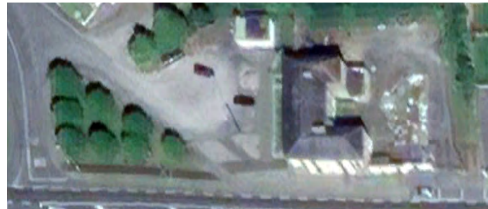
Aerial image (2022) showing the extents of hard surfacing at the Courthouse.
