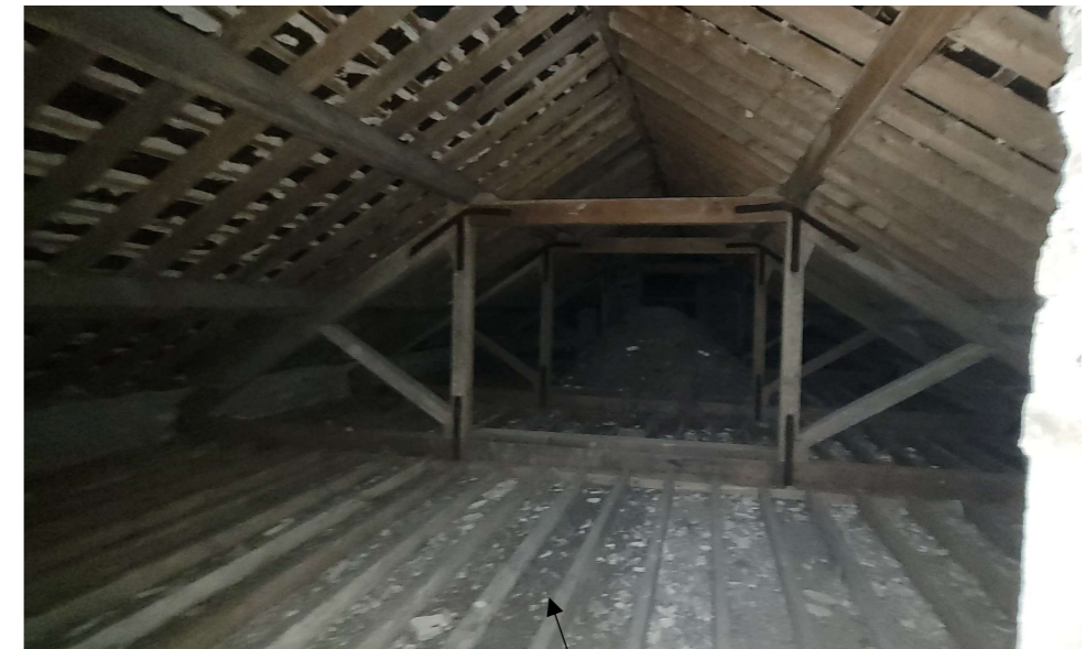
Attic - existing condition
