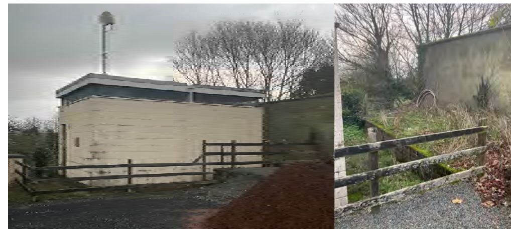
Telecommunications building and the dead space to its rear
