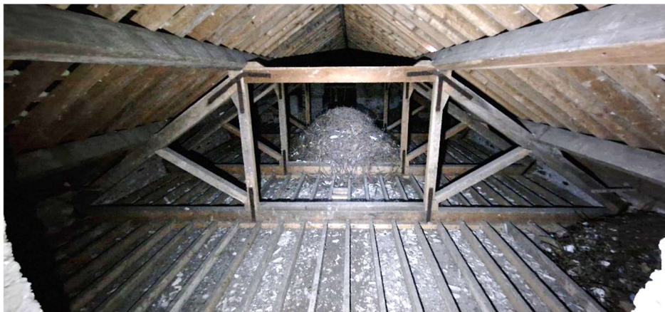
Figure 9 – Queen post trussed roof over courtroom
