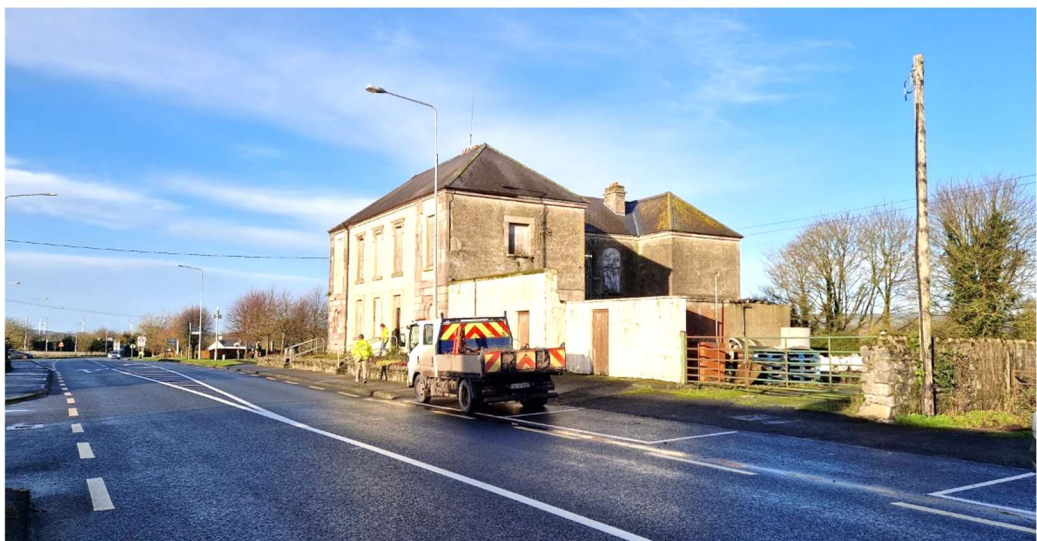
Figure 3: East elevation of courthouse with stored materials visible in foreground
