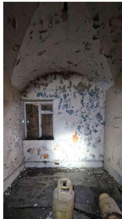
Figure 19 – Room GF-4 in north wing
