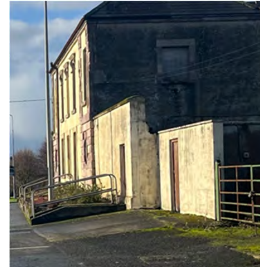
Walls to the east of the Courthouse
