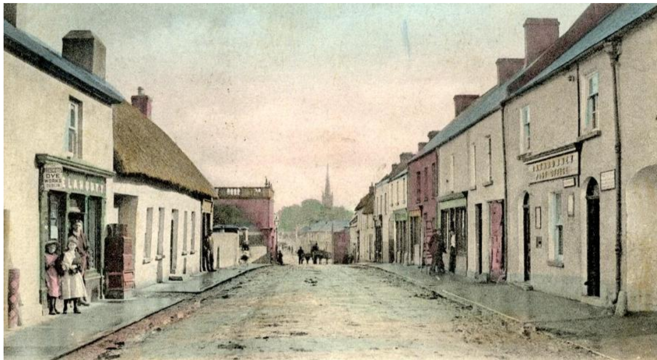
Historic view of Main Street and St. Andrew's church tower
