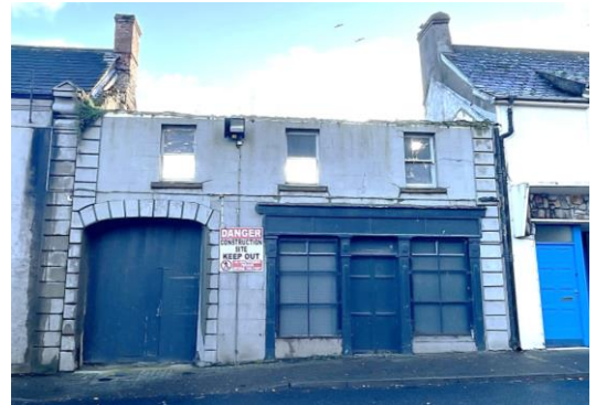
Derelict heritage building
