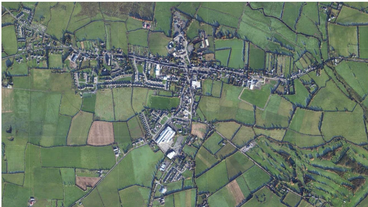
Aerial View of Rathdowney
