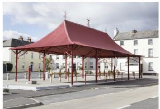
Stradbally Market House
