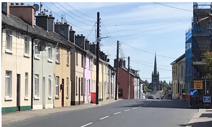
Overhead cables, Main Street
