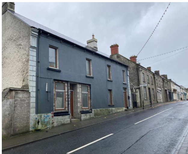
Vacant buildings / refurbishments at Main Street
