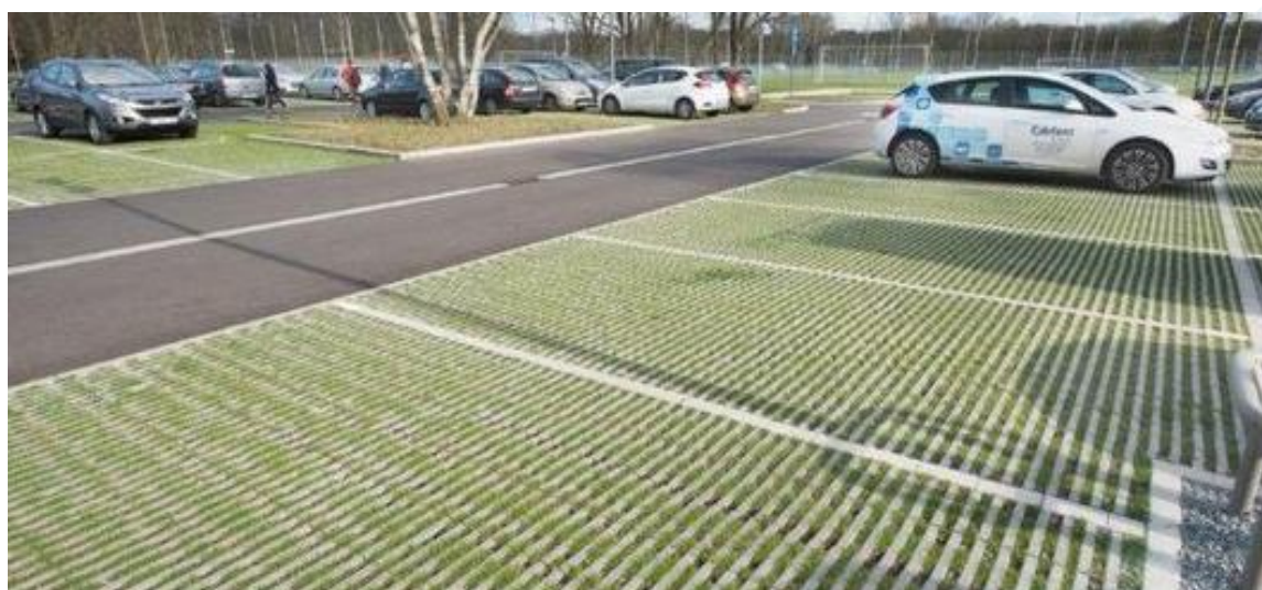
Figure 3.2 Precedent image of a car park with permeable grass paving
