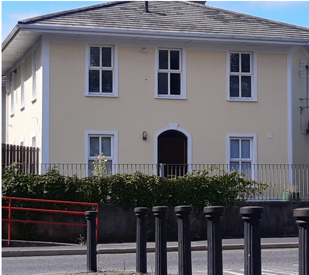
Existing apartment at Riverview development in Portlaoise
