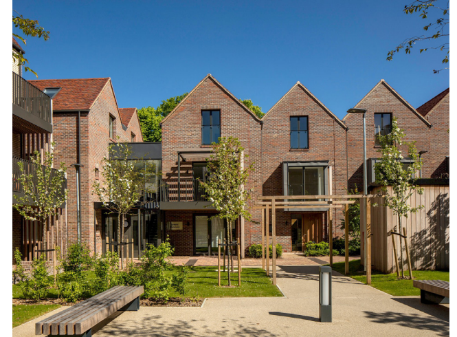
Residential development with shared community space and a focus on green infrastructure
