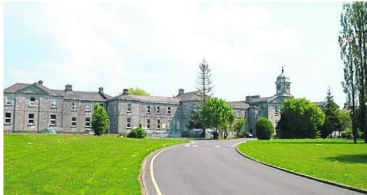
Plate 19: Saint Fintans Hospital Complex, Dublin Road, Portlaoise
