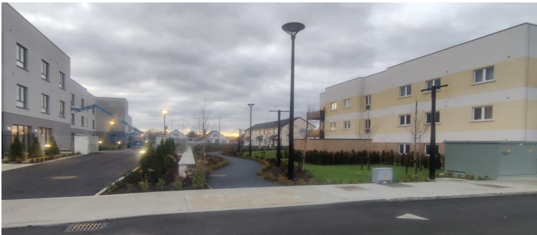
Plate 2: New housing development on former Granary site, Portlaoise town centre
