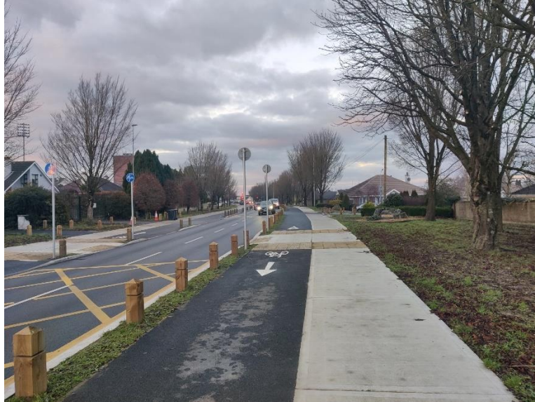
Plate 15: Provision of cycleway and reduction of road width on Abbeyleix Road N77.
