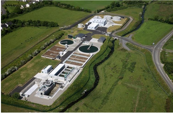
Plate 12: Uisce Eireann Treatment Plant at Ridge Road
