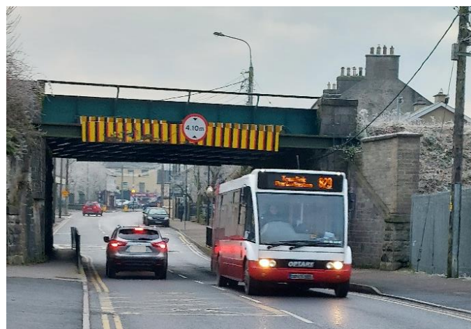
Figure 14-2 Bus service travelling under the railway bridge on Coote Street. Source: DBFL.
