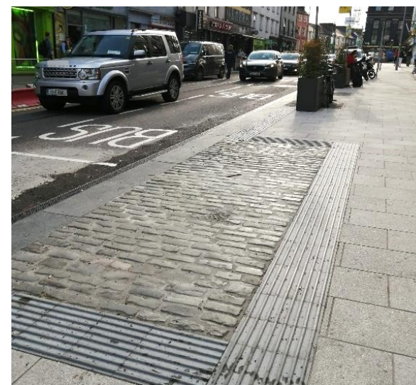
Figure 16-2: Alternatives to on-street car parking. (Top) Covid mobility measures in Dungarvan where seating areas for restaurants and cafes and landscaping replaced parking spaces. (Bottom) Newly constructed dual-purpose loading bay in Cork. Photos: J. Egan
