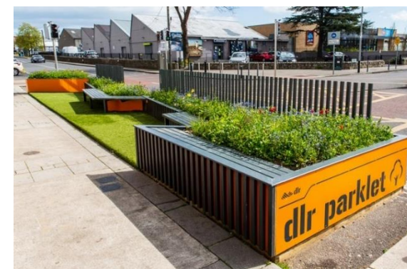
Figure 17-9 SuDS in the form of a Parklet along Sallynoggin Rd in Dún Laoghaire. Source: Dún Laoghaire-Rathdown County Council.
