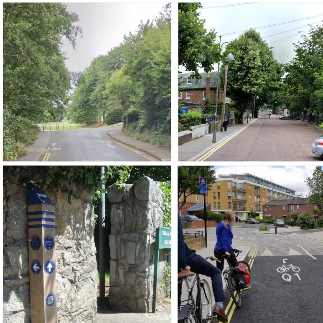
Figure 12-8 Varieties of Quietways and Wayfinding. (Top Left): Ballybrack/Mangala Greenway in Cork that uses quiet streets and a greenway to deliver local connectivity. (Top Right): Mardyke Walk, Cork, has red paving and a 30km/h speed limit to provide a Quietstreet. (Bottom Left): Wayfinding for Safe Routes to School in Dún Laoghaire Rathdown. (Bottom Right): Marked Quietways in London. Sources: Streetview, NTA Cycle Design Manual and DBFL.
