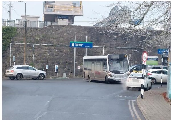
Figure 14-7 Cars, a taxi and a bus all stopped outside the Railway Station. Source: DBFL.
