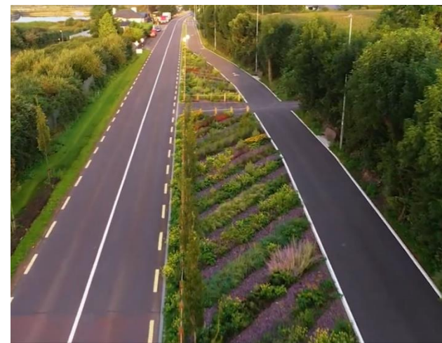
Figure 17-8 The Dunkettle to Carrigtwohill Cycleway Scheme, with SuDS in the form of a pollinator corridor. Source: Cork County Council.
