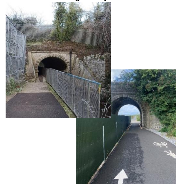
Figure 12-6 (Top) Existing section of the Triogue Way. (Bottom) A section of the Tralee to Fenit Greenway, illustrating an opportunity for improved security along the Triogue Way. Source: DBFL.
