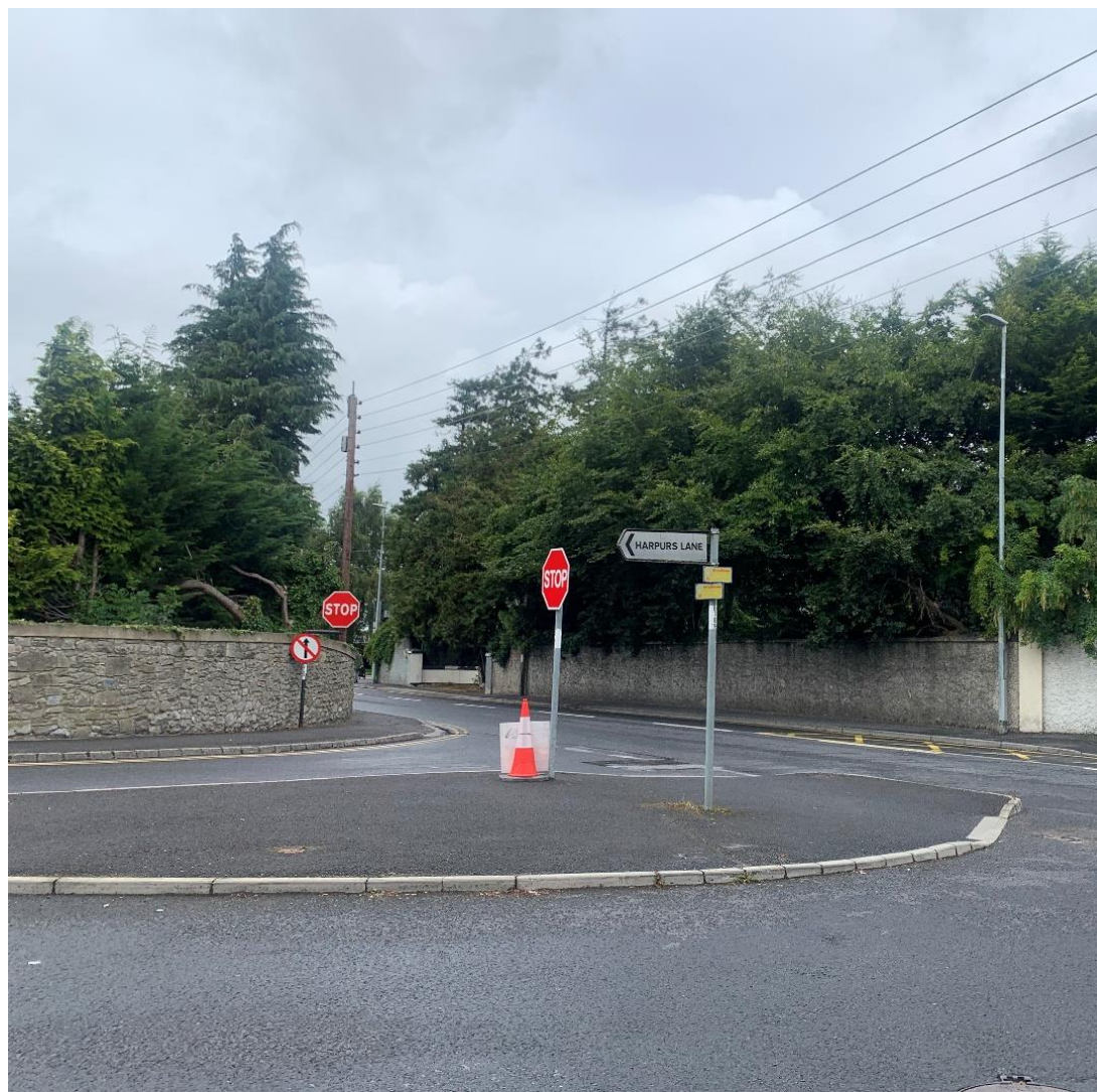
Figure 10-1 The junction of Harpur's Lane and Mountmellick Road typifies some junctions in Portlaoise with wide corner radii, excessive turning lanes and little provision for pedestrians or cyclists. Source: DBFL.
