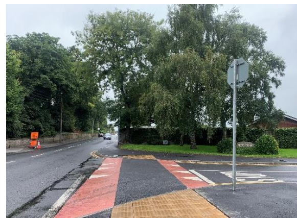
Figure 6-8 A junction tightening at Beechfield completed with NTA funding. Source: DBFL.
