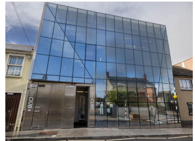
Figure 20-1 The CUBE Low Carbon Centre of Excellence in Portlaoise offers meeting rooms for local businesses, as well as consultancy and training service. Photo: Alf Harvey.
