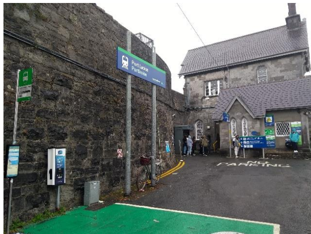
Figure 14-1 The entrance to Portlaoise Railway Station, which has EV Charging points, a bus stop and bicycle parking. Source: DBFL.
