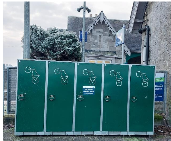
Figure 14-5 Bike lockers at Portlaoise Railway Station. Source: DBFL.
